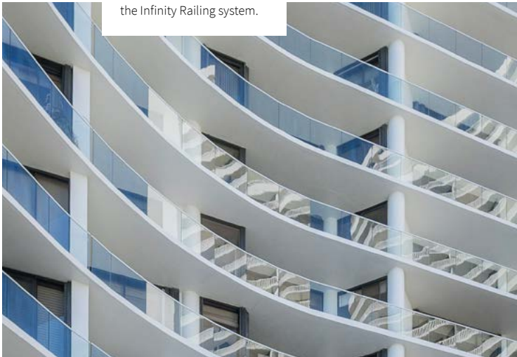
Before & after: Replacement of the railing balustrade by Poma with the Infinity Railing system.
